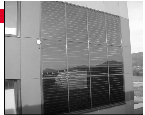
Test façade with a 25 m 2 collector on a brick office building in St. Veit, Austria.
