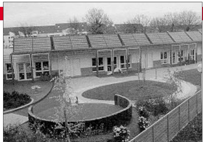
A preschool in Bretagne that is equipped with a medium-sized centralized solar water plant.
