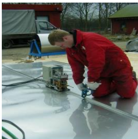
Figure 5. Induction welding of a stainless-steel liner [5]
