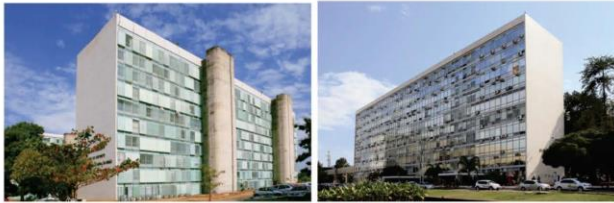
Figure 2. West and East façades of the building.
