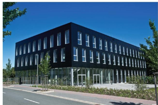
Figure 1. DIAL Headquarter Lüdenscheid. The windows are floor-to-ceiling and lintel-free.
