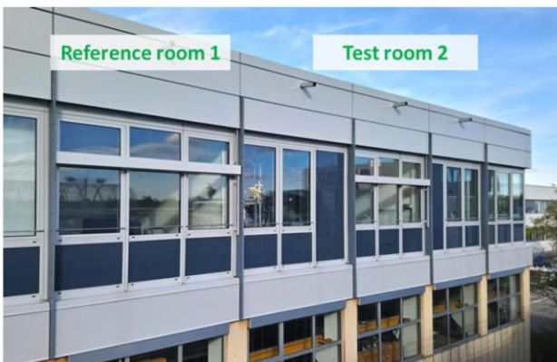
Figure 4. An exterior view of the lab. The façades of both the reference and test room can be seen in the picture.
