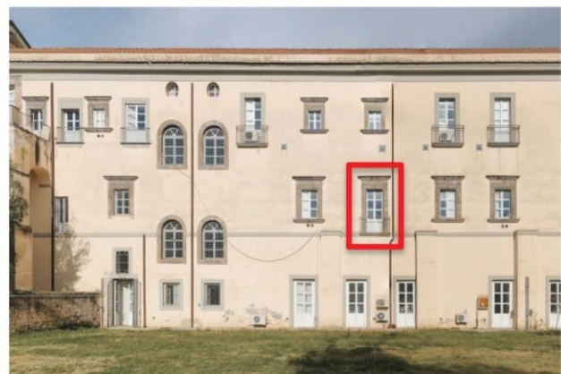
Figure 1. External view of the Abazia San Lorenzo ad Septimum façade.
