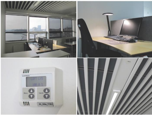
Figure 2. Lighting and solar control in typical office space (04.103) at Navitas.
