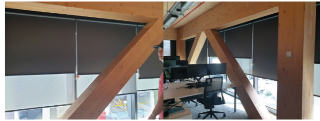
Figure 11. Real outcomes from conducting a POE survey, where glare was reported by a significant number of occupants. Additional blinds were installed with lower VLT (<10%), to deliver a double roller strategy for increase control of daylighting.
