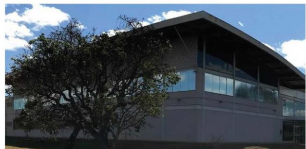
Figure 1. Office building at the University of Brasilia campus.
