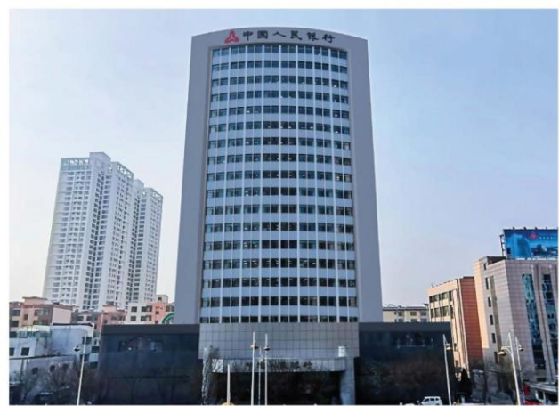
Figure 1. The Xining Central Sub-branch of the People's Bank of China.
