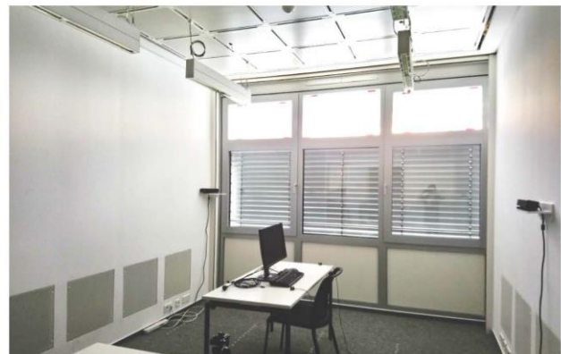
Figure 1. The lab room seen from the inside. The micro-optical panels are placed on the top part of the windows and provide a soft daylight illumination deep in the room.
