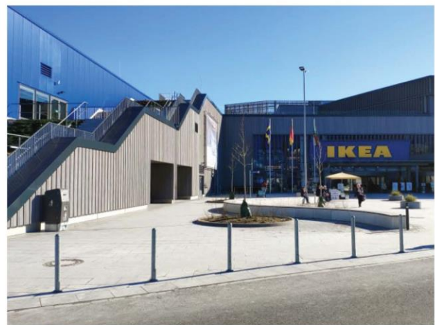
Figure 1. The IKEA shop in Kaarst as seen from the outside. The windows in the living room exhibition area can be seen at the top of the first flight of stairs.
