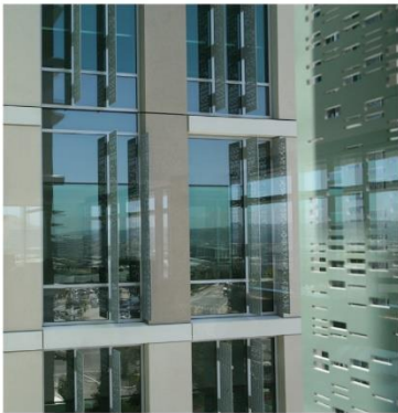
Figure 5. Exterior vertical fins on east and west facades.
