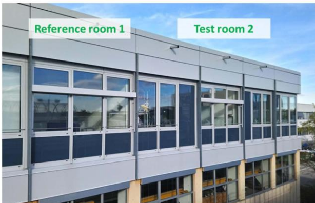
Figure 2. An exterior view of the lab. The facades of both the reference and test room can be seen in the picture.
