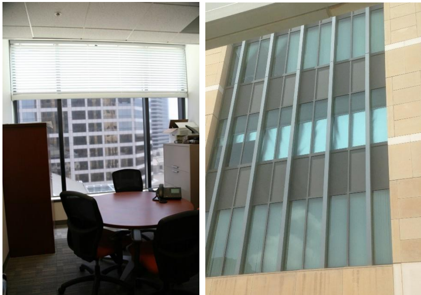
Figure 8. Indoor (left) and outdoor (right) view of the dual-zone shades at US DualZoneShade, Oakland, CA.
