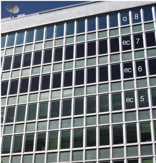
Figure 2. Outdoor view of the south façade with electrochromic (ec) and original (o) windows.
