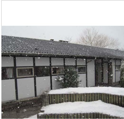
Façade facing playground - Before renovation
