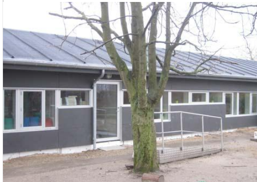
Façade facing garden - After renovation
