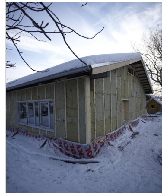
Above: Old insulation has been removed and new windows have been installed Below: New insulation has been added
