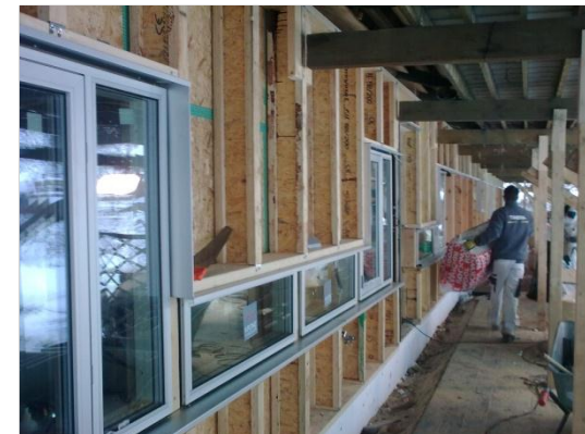
Above: Old insulation has been removed and new windows have been installed Below: New insulation has been added
