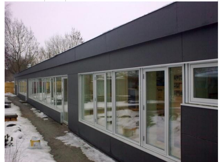
Right: Facade facing the playground after renovation. The new facade requires little/no maintenance.
