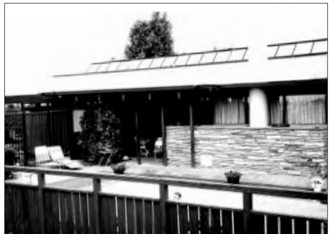
Figure 2: A Colorado residence with a solar air system still in service 40 years after installation.
