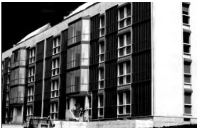
Figure 4: The Marostica apartments in Italy with a Type 2 solar air system.
