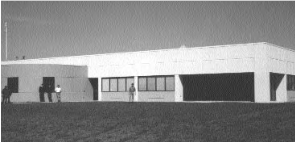
The Energy Resource Station (ERS) test facility in Ankeny, Iowa. ERS has 4 sets of matched test rooms and a sophisticated HVAC system to create laboratory quality test data for purposes of empirical validation of building energy analysis tools.
